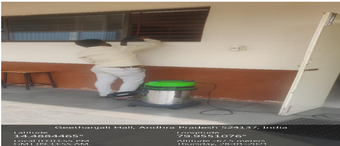
Maintenance of Window Grills
