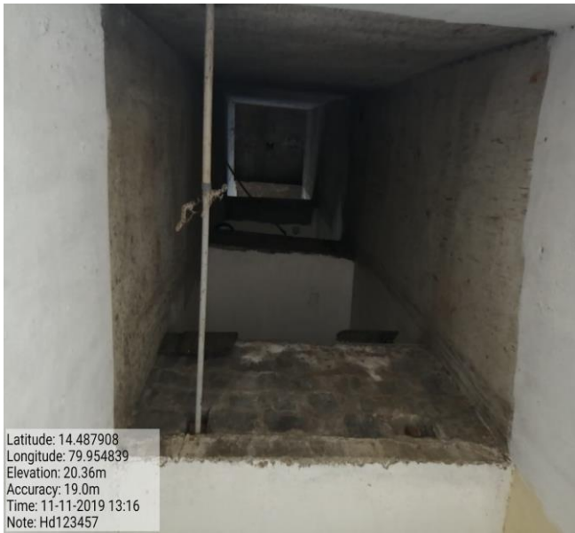
Fig:- Provision for Lift
